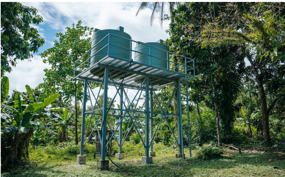
Caption: The two 10,000L water tanks in Qurasae, Western Province, has helped addressed the community's greatest problem of having source water from brackish water.
