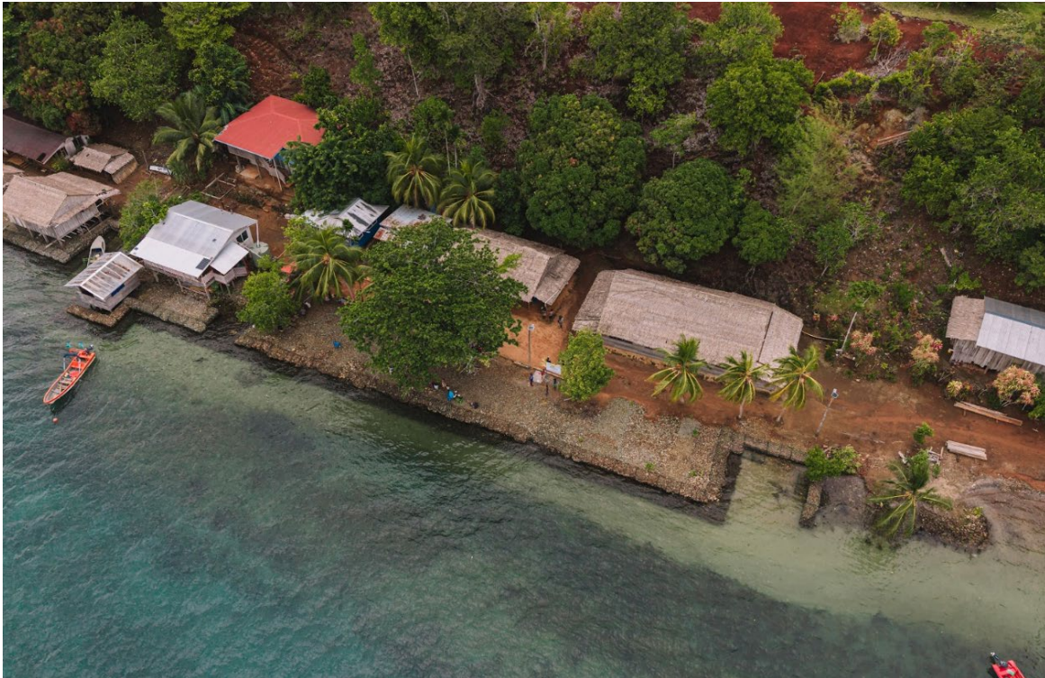
Caption: The new seawall in Horara, Isabel Province is protecting the community from coastal erosion and rising sea levels, allowing the village to replant gardens, secure properties, and return to the homes they have lived in for generations.
